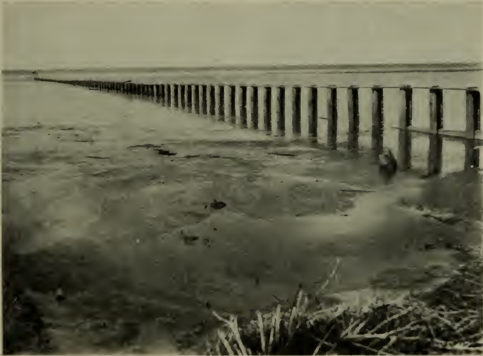
Fig. 2. Partially Constructed Groyne of Reinforced Concrete. COAST PRESERVATION IN BRITISH GUIANA.
